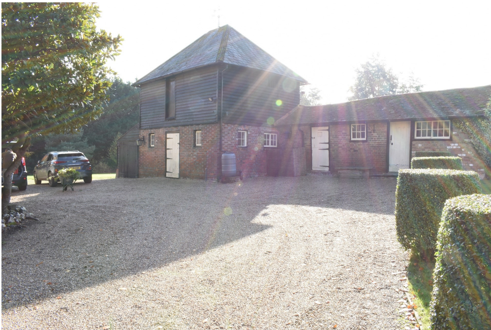
Plate 11: View across the yard towards the proposed development area showing the barn and stables (facing S)
